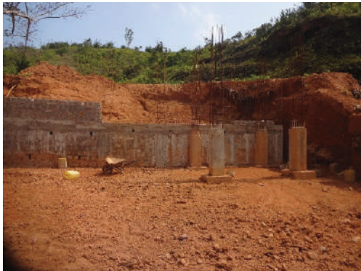
Civil foundations for erection of feed bunker and new plant shed
