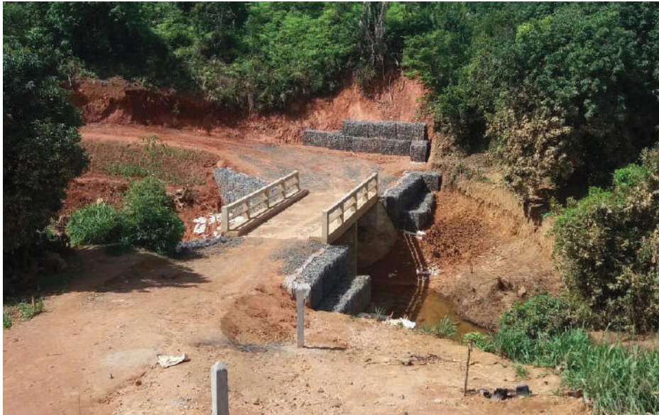
Newly constructed 11m long bridge connecting the site to the national highway
