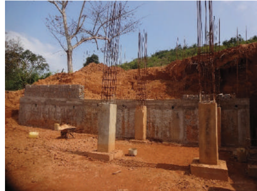
Civil foundations for erection of feed bunker and new plant shed
