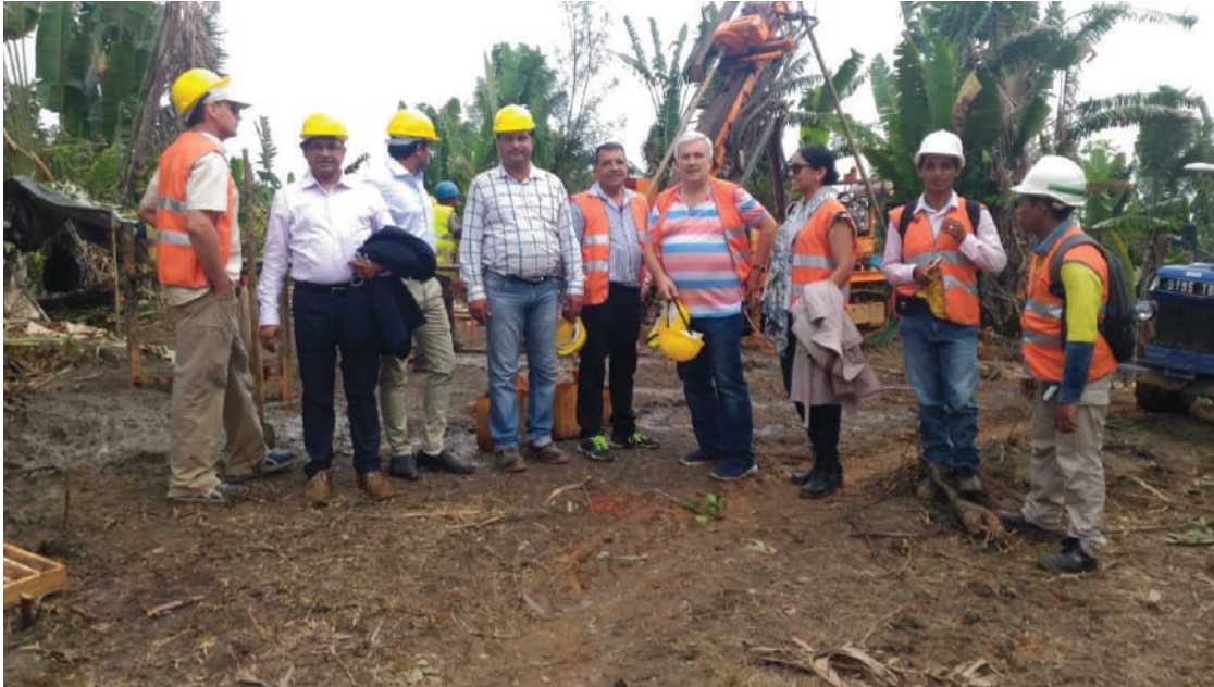
Visit of auditors to drill pad where drilling was ongoing
