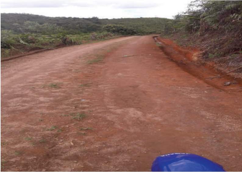
Newly-improved approach road
