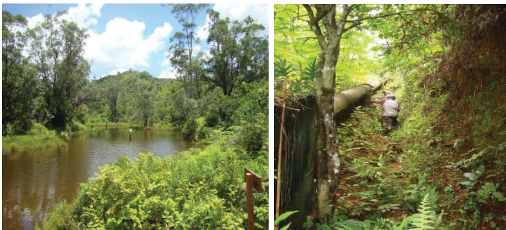
Reservoir and pipeline for Hydro power plant
