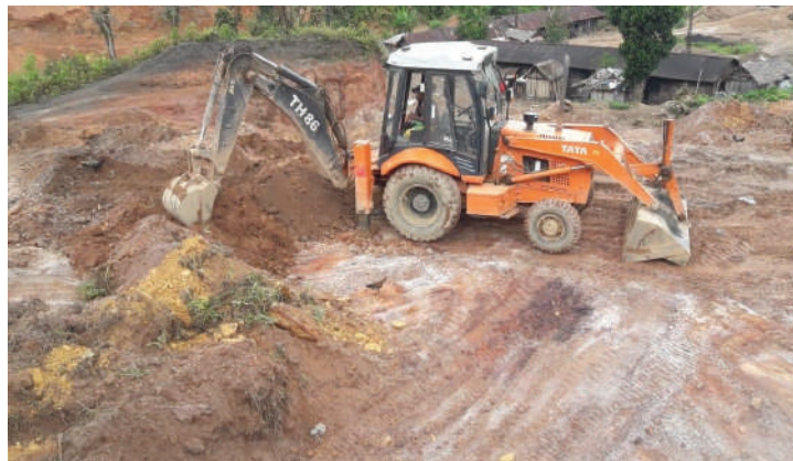
First set of versatile small earthmover equipment commissioned.
